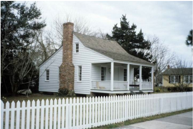
5. Chimney or Fireplace.
