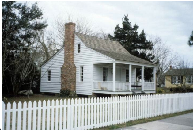
5. Chimney or Fireplace.
