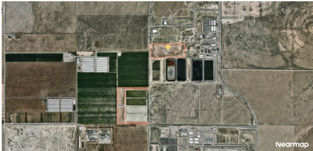
Figure 5. Public works subunit.
