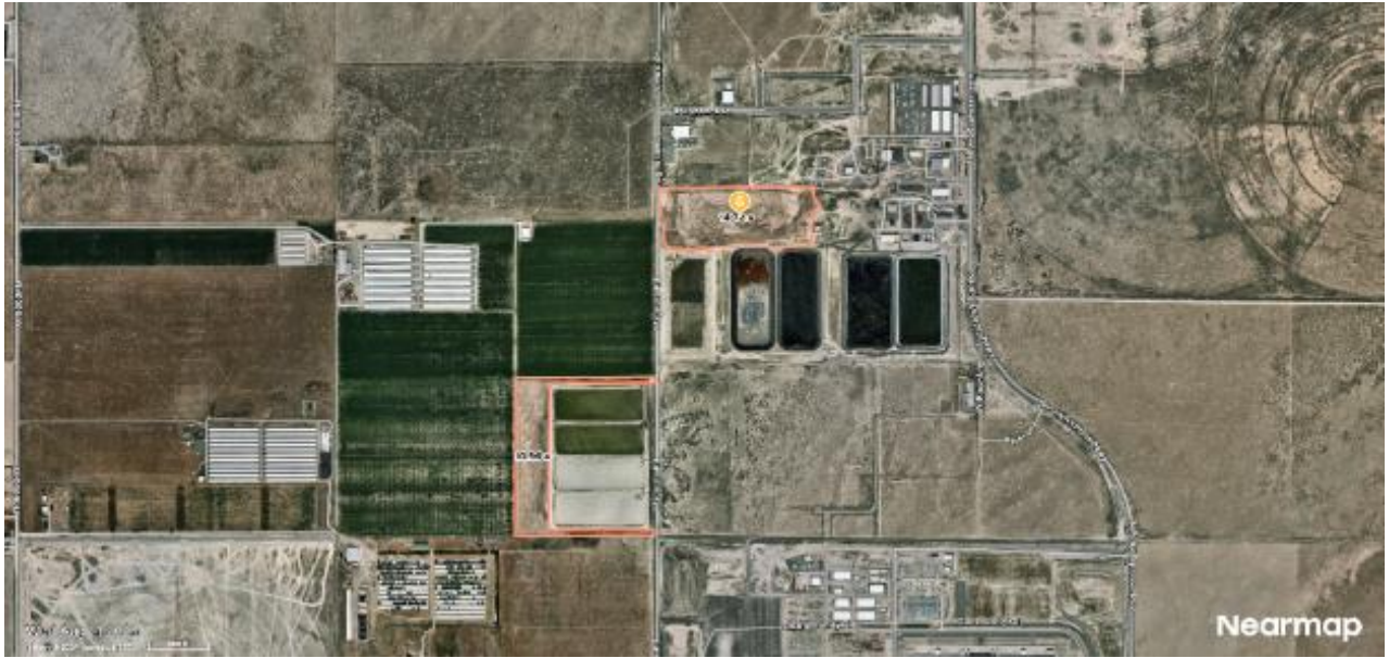
Figure 5. Public works subunit.
