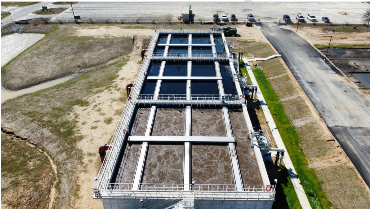
Figure 6. AquaNereda® Aerobic Granular Sludge System (Aqua-Aerobic Systems Inc.)
