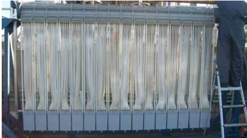
Figure 12. MFS rack during installation
