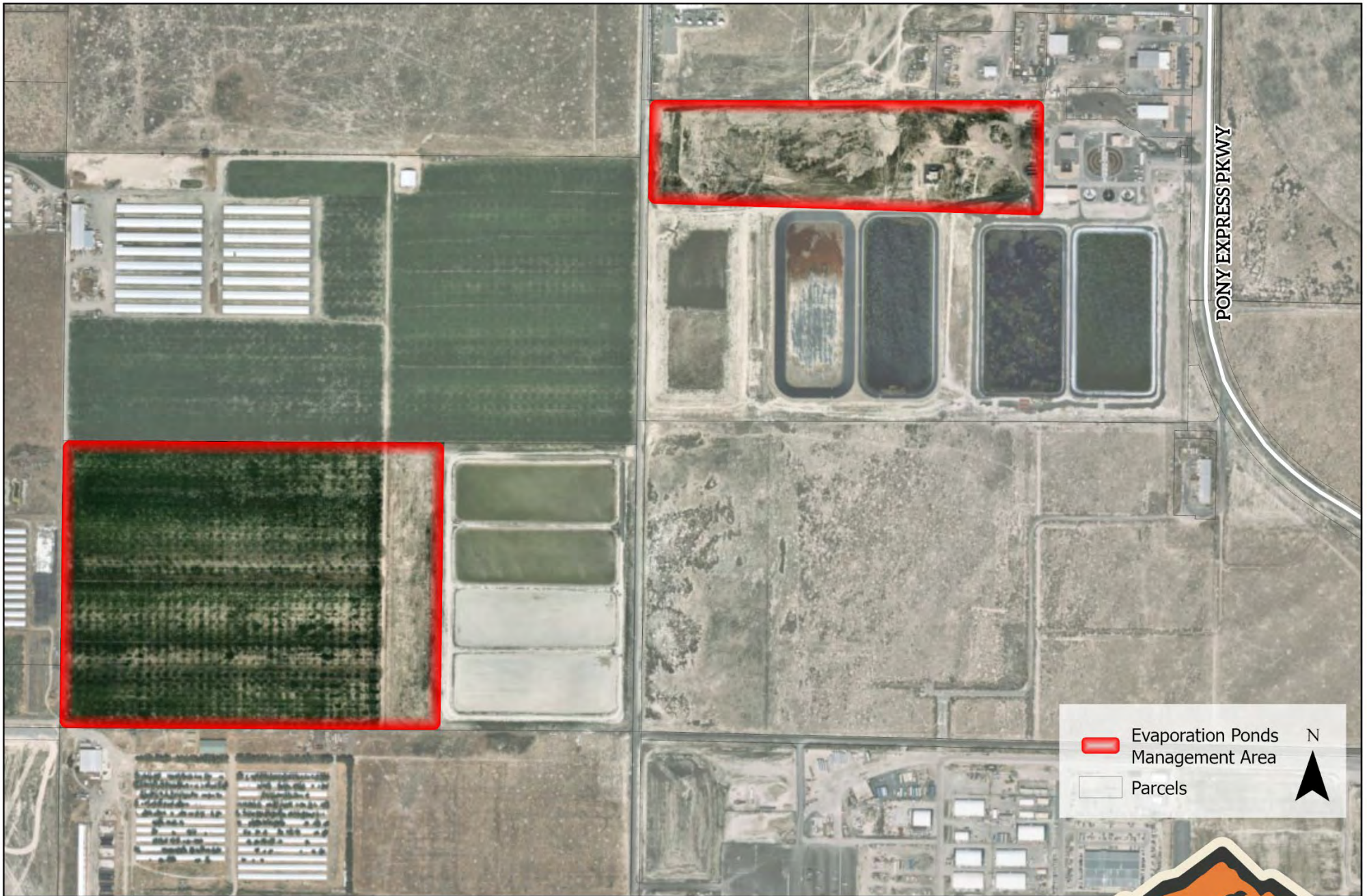
Figure 16. Evaporation Ponds Utility Management Area
