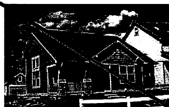
Examples of poor building massing and scale.
