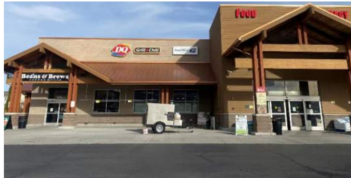
Required: Clearly identifiable covered entry
