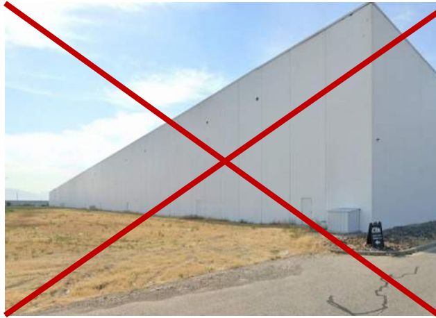
Not permitted due to lack of building articulation
