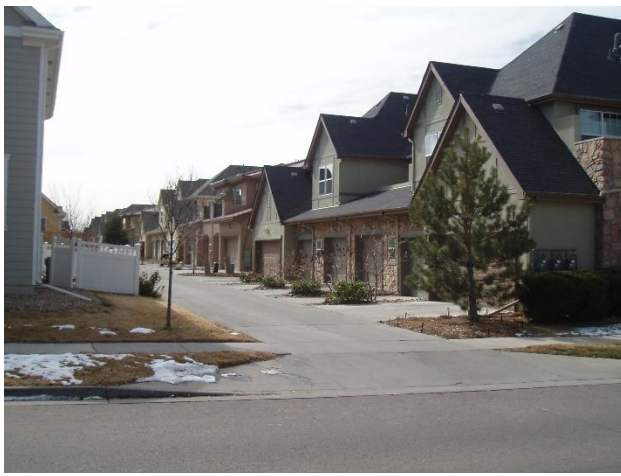
Garages accessed by private service drive
