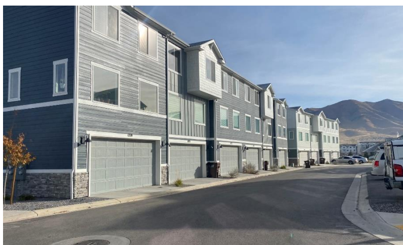
Garages accessed by private service drive
