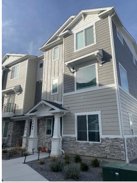
Multifamily unit entry defined with covered porch
