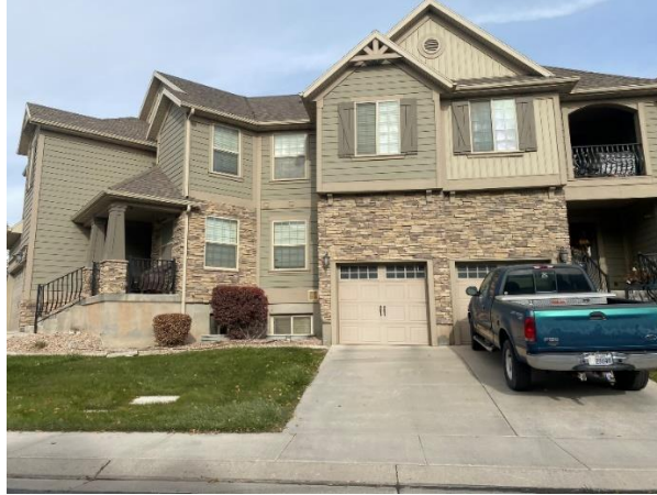
Decorative parapets and multiple roof planes/projections
