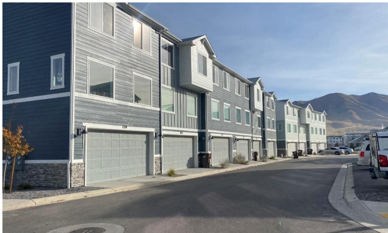
Garages accessed by private service drive
