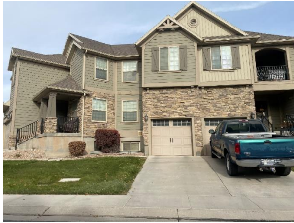
Decorative parapets and multiple roof planes/projections
