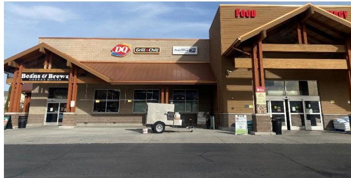
Required: Clearly identifiable covered entry
