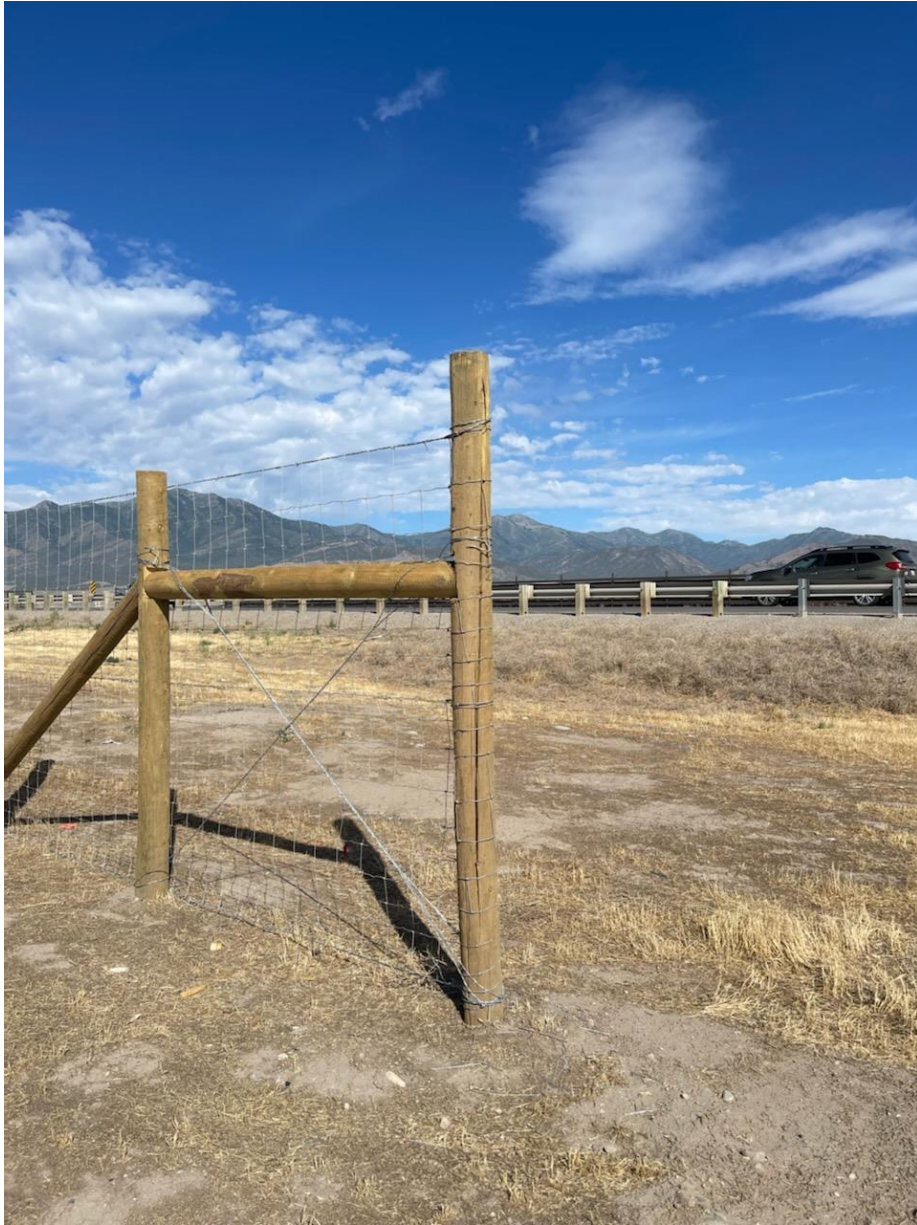
Figure 2, (left) picture of the wildlife gate post and opening on the south side of SR 73 to the west. Figure 3 (right) picture of the wildlife gate post and opening south of SR 73. The opening between this post is 45'.
