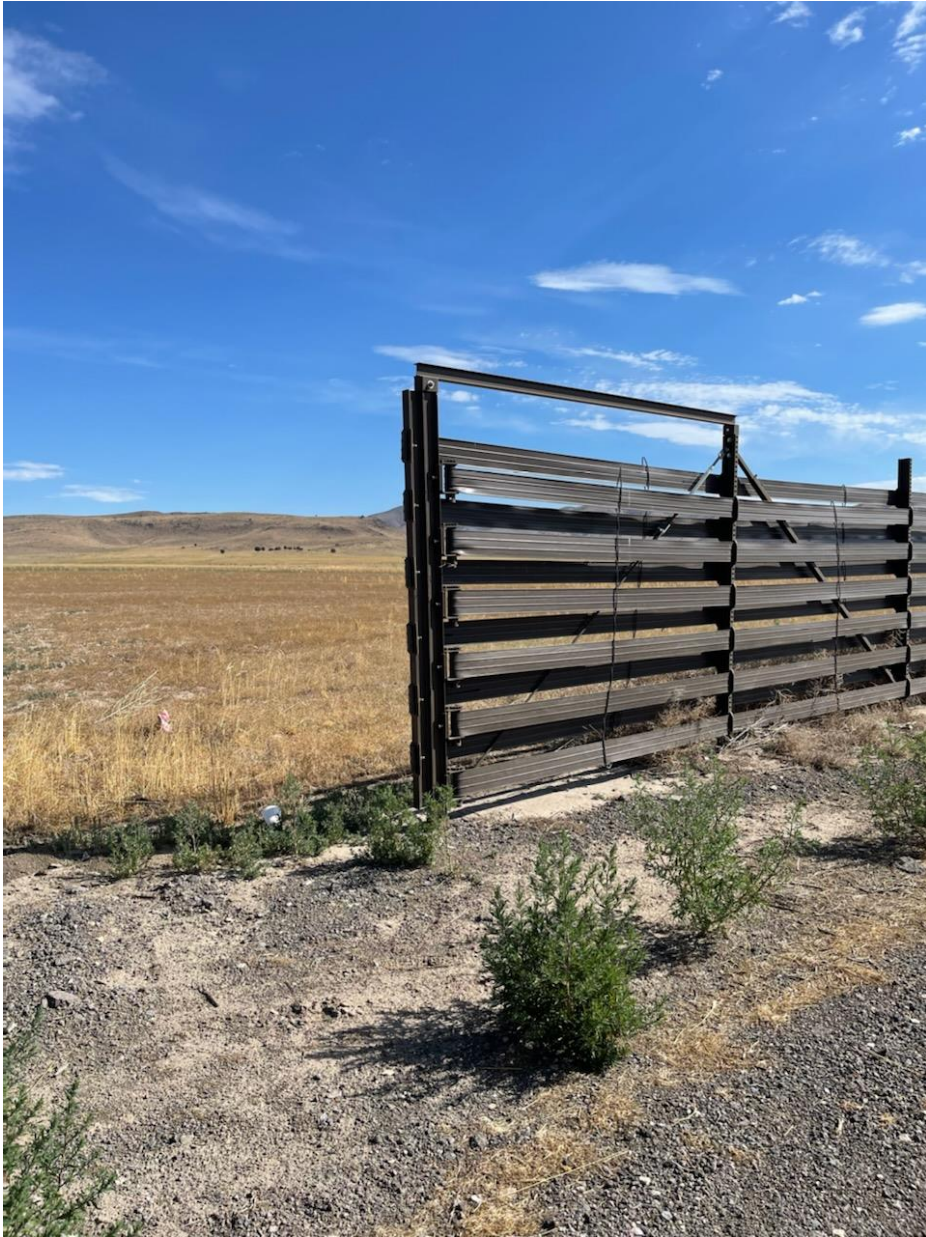
Figure 4, (left) picture of the snow fence gate post and opening on the north side of SR 73 to the west. Figure 5 (right) picture of the snow fence gate post and opening north of SR 73. Opening between these two posts is 69'.
