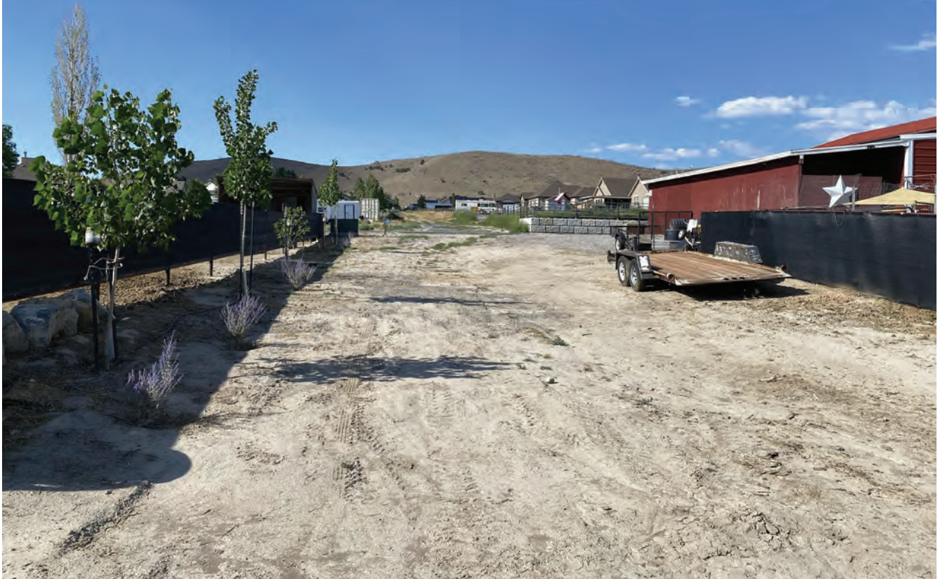
East Trail Looking Southeast over Retention Pond
