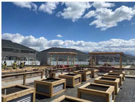
Garden Fencing - 36" wood frame with wire mesh paneling. Garden Boxes with wood frame and corrugated metal panels.
