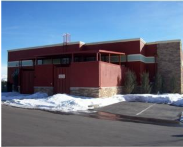
Screening for mechanical equipment matches building in material and color
