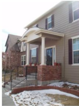
Multifamily unit entry defined with covered porch
