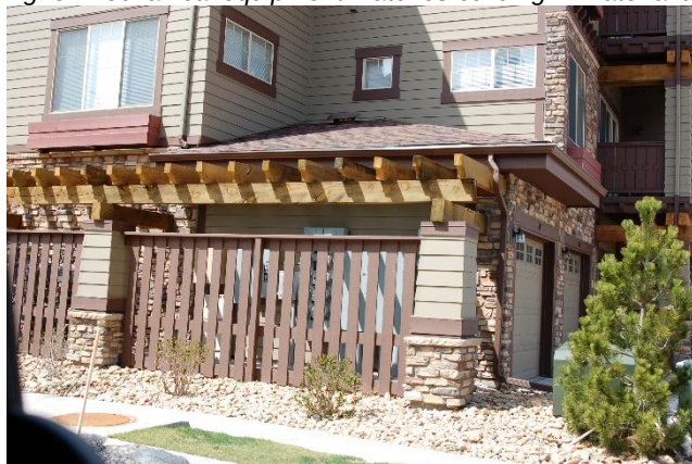
Screening for mechanical equipment matches building in material and color
