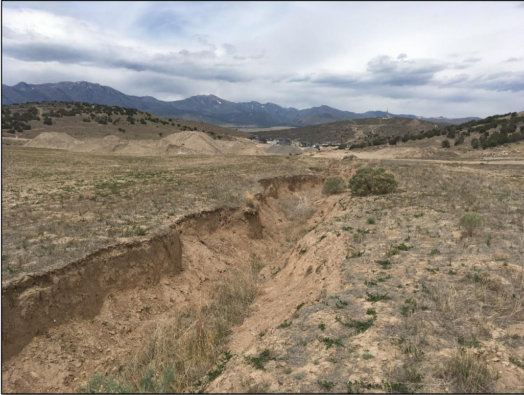
Drainage Ditch on Subject
