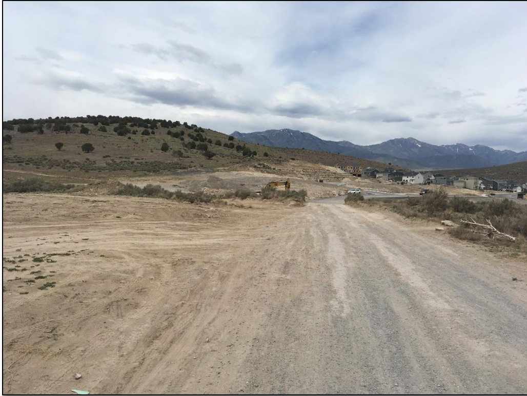
Northwesterly View Along Hidden Valley Parkway
