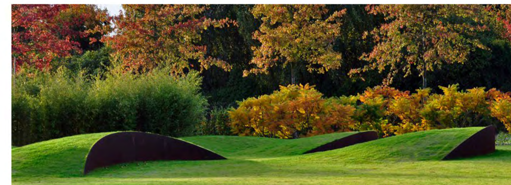
LAWN BERM CUT WITH RETAINING WALL
