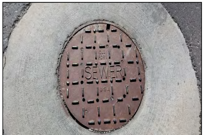
Picture 12 – Sewer lines were observed along North Lake Mountain Road and Eagle Mountain Boulevard.
