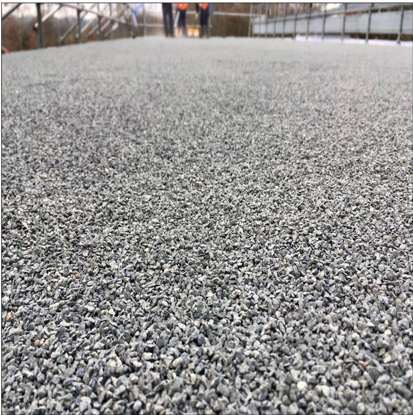
GRAVEL BALLAST - ENTRY CANOPY
