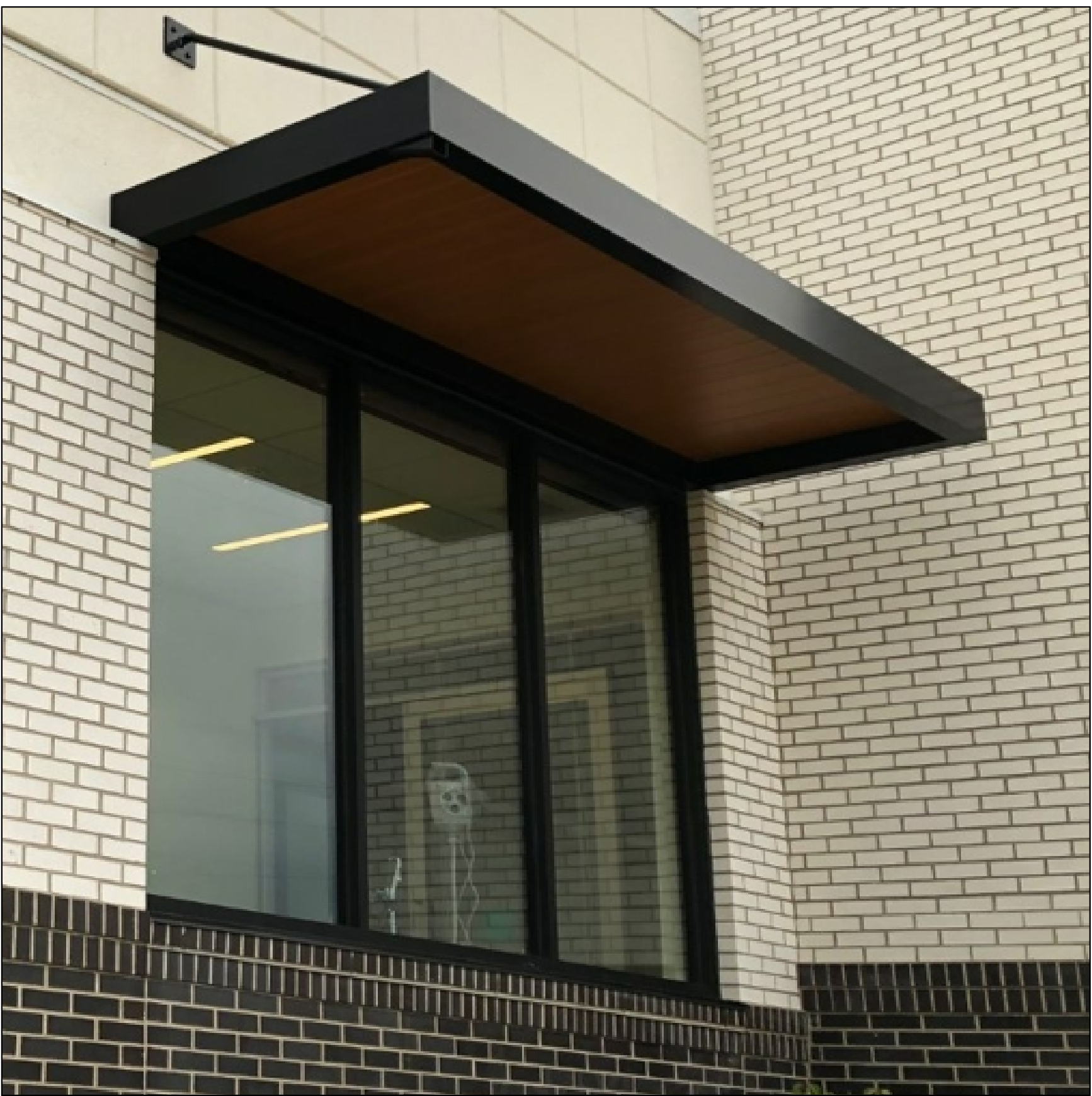
ENTRY CANOPY - WOOD SOFFIT
