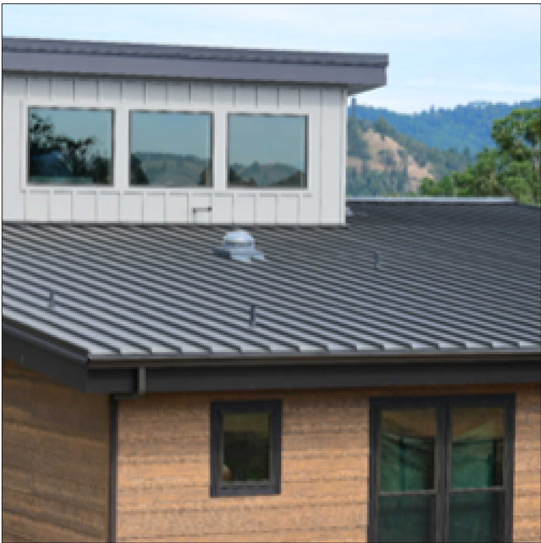
STANDING SEAM METAL ROOF
